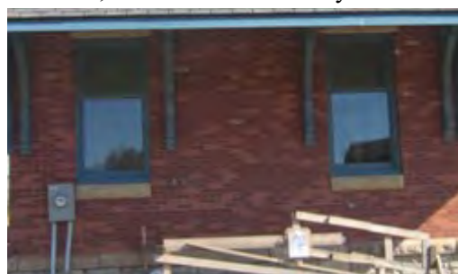
2019 South wall with added recycled brick
