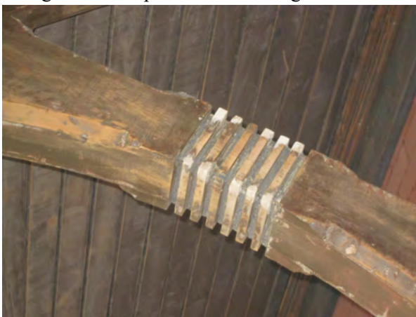
Repair: Some corners of bracket slots were missing, but repaired. Nail holes were filled. Wood in excellent condition.
