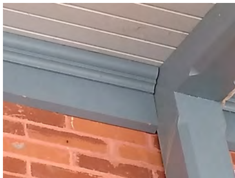
2019 New cornice board on south wall
