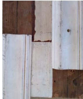
Mock up of crown moulding placing two pieces of moulding on each side of the 7" board.
