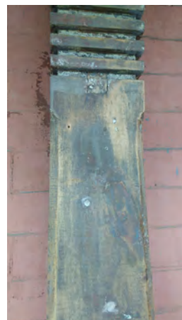
Removal of paint revealed original color.
