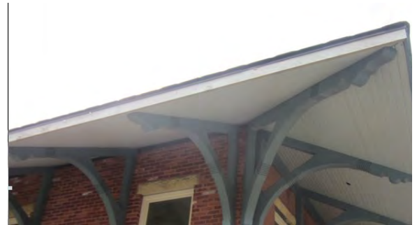
2019 New soffit on left; original on right
