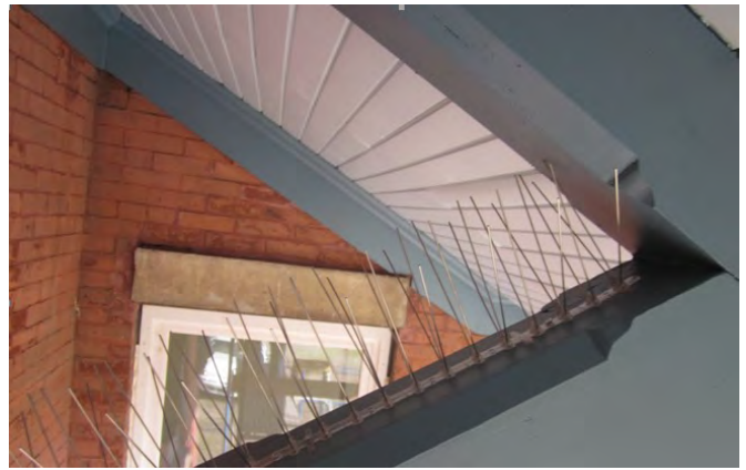
All old paint removed from original soffit v-board; painted with a very light shade of the gray-blue found under light mounting.
