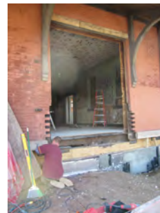
2019 Retained location of 1944 opening, lintel and brackets.
