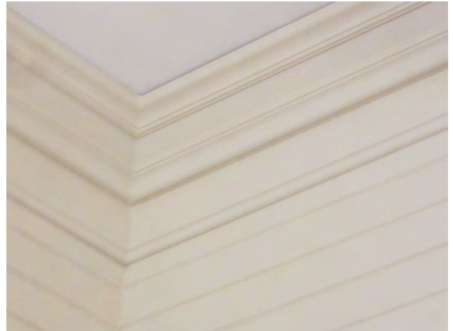
2019: New crown moulding using of same dimensions of original.
