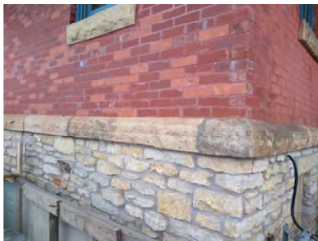
Original stone added to south wall (left) Original stone in place (right)
