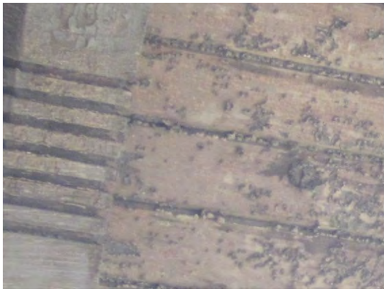
No color could be discerned on the old soffit paint crumbles in the v-board joints and board.
