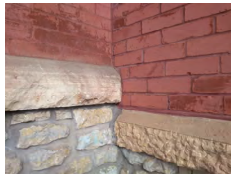
Original stone in place on main room (left) Recycled stone on baggage room bump-out (right)
