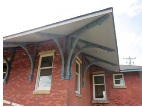
2019 Four new brackets on south(left) and two original on east (right).
