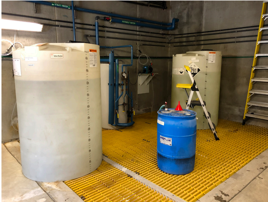
Figure 5. Odor Scrubber Chemical Storage (Containment under Bisulfate Tank Is Inadequate)
