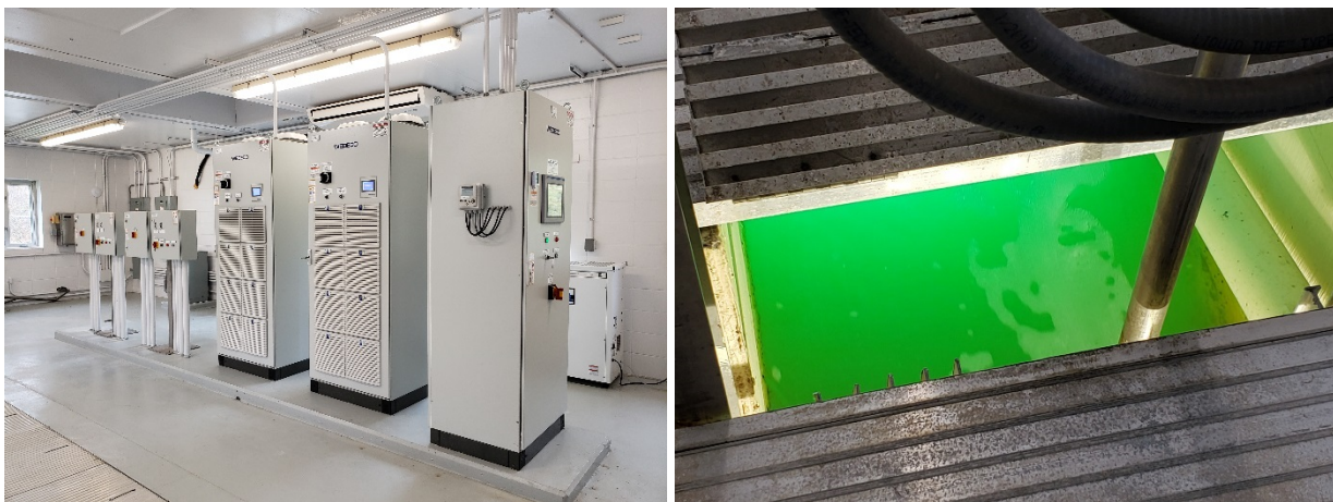
Figure 4. Left: UV Controls. Right: UV Light in Water.
