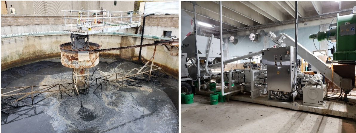
Figure 5. Left: Solids Storage in Decommissioned Clarifier. Right: Temporary Dewatering, Lime Addition, and Reactor.
