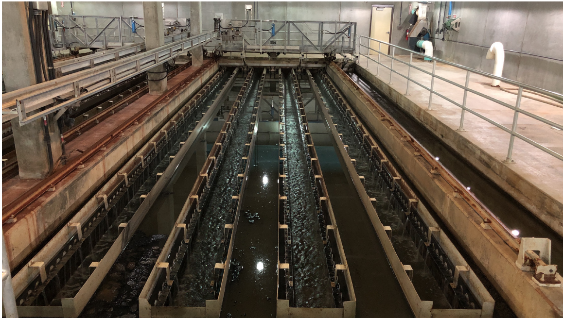
Figure 3. Primary Clarifier (In Service)
