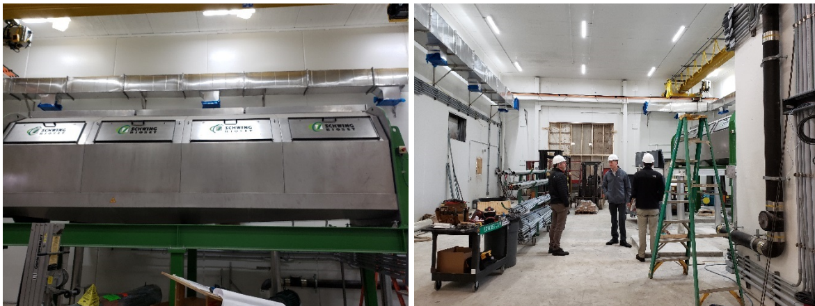
Figure 6. Left: Newly Installed Screw Press for Solids Dewatering. Right: Newly Renovated (Still in Process) Solids Dewatering Room.
