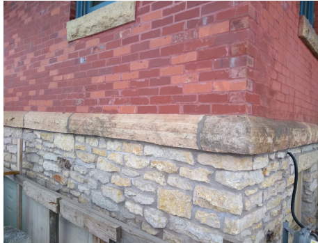
Original stone added to south wall (left) Original stone in place (right)
