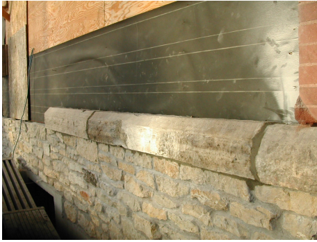
Original water table from baggage room bump-out added to new south wall.
