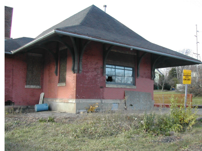
1944 Conversion: Two windows were replaced with one picture window
