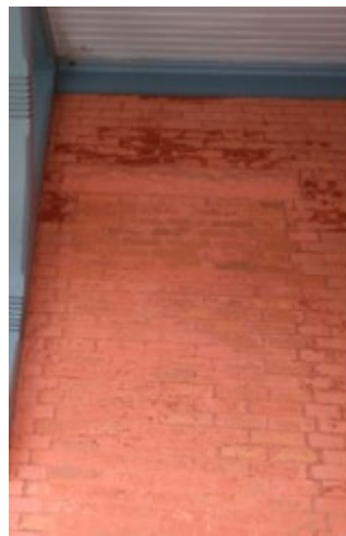
One of two lintels painted over when doors removed and openings bricked over in the 1910 addition of restrooms.
