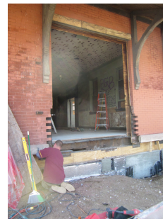
2019 Retained location of 1944 opening, lintel and brackets.
