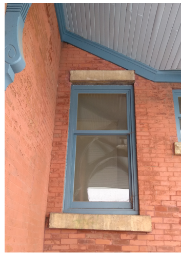
One of two 1910 windows with smooth concrete lintels and sills in the added restrooms in the former baggage room.
