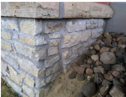
Exposed limestone in gap between wall and east side steps leading from the sidewalk to the platform. A similar gap is on the west side between the steps and platform.
