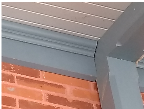
2019 New cornice board on south wall
