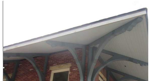
2019 New soffit on left; original on right
