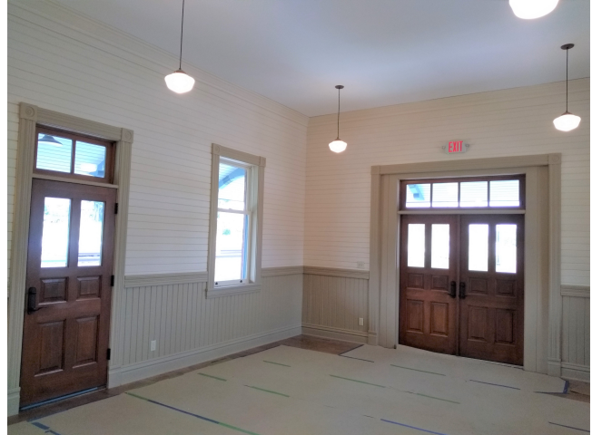
2018: Ceiling raised 2' to original position on original rafters.
