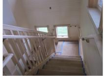
2019: Carpenter installed maple stairway to the basement; wood finish will be added to match new flooring.
