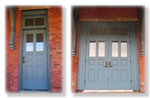
The doors and transoms were custom ordered using the original 1888 blueprint design; the double doors will open onto the floor of the pavilion.
