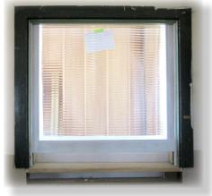
In 1944, two separate ticket windows (one for women and one for men) were removed and replaced with one window. The unique glass was broken sometime after the depot closed. A volunteer found glass that was similar and replaced the window. The iron weights that lower and raise the window remain in place.
