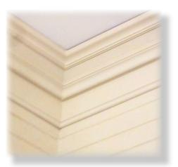
Close-up of the reconstructed four-piece crown moulding. The unpainted V-board at the top of the walls indicated an original wide crown moulding removed when the ceiling was lowered in 1944. A portion of the original crown moulding was found in the attic providing an additional clue about the size and the design.
