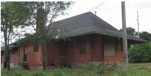
East side (Hwy. #3): Reflects 1911 bump-out modification of baggage room into bathrooms and boiler room.
