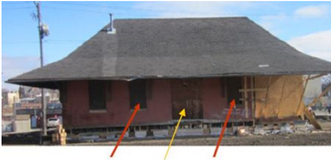
West side (track side): red arrows = 1944 windows added in 1888 door openings (now restored); yellow arrow = 1944 addition of doors after removal of 1888 station master bay (now restored).
