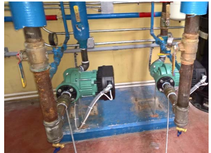
WWTP Boiler Pumps
