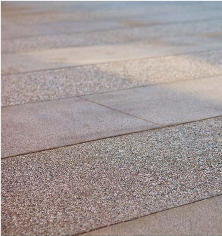
topcast concrete - saw-cut edges
