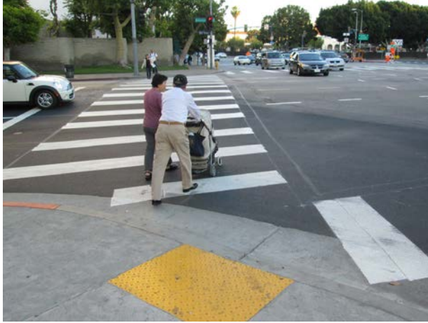
Not recommended: Diagonal curb ramp configuration.
