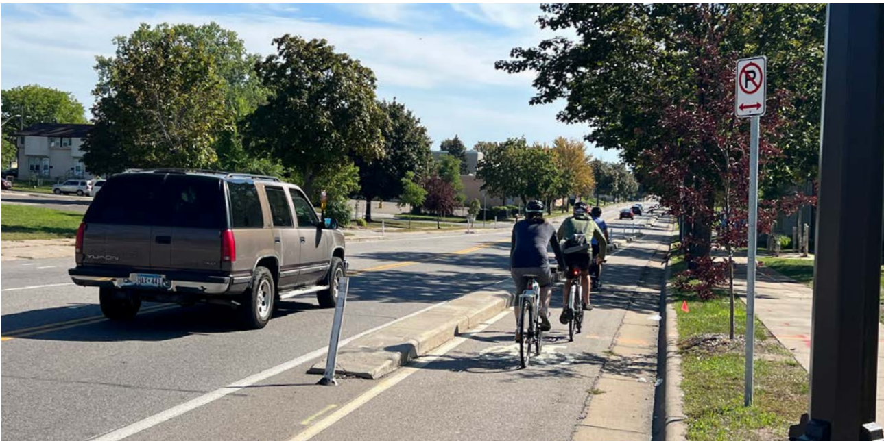
One way separated bikeway example with concrete bike buffer in Minneapolis
