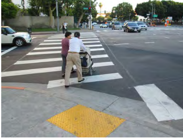
Not recommended: Diagonal curb ramp configuration.
