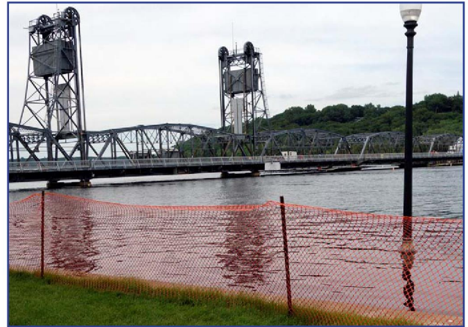
Stillwater Lift Bridge, 2018, during renovation as a pedestrian and bicycle path, and a foreground interpretive panel on bridge history and operation.
