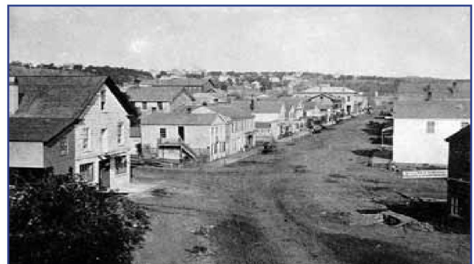
Main Street looking north in 1870. MNHS
