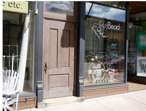
Central entry with cast-iron columns, 2016.
