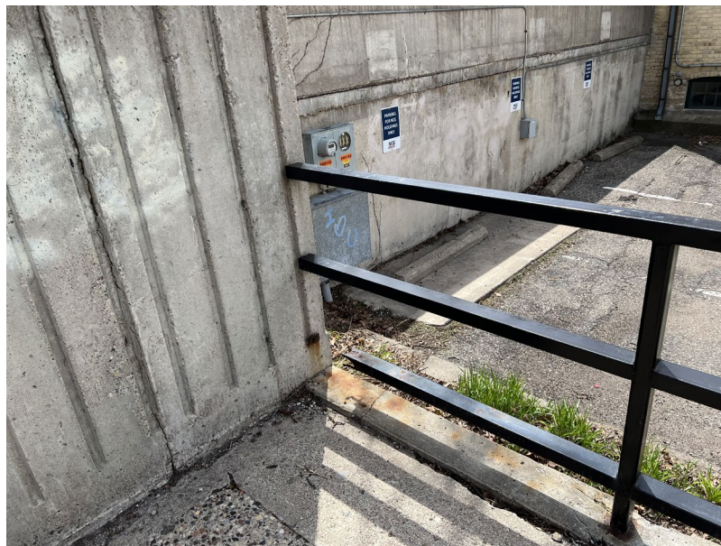
Broken railing
