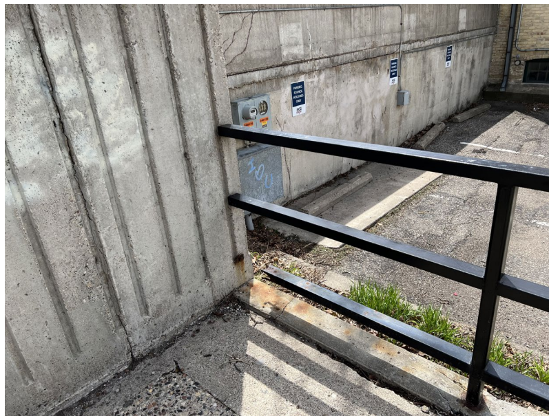
Broken railing
