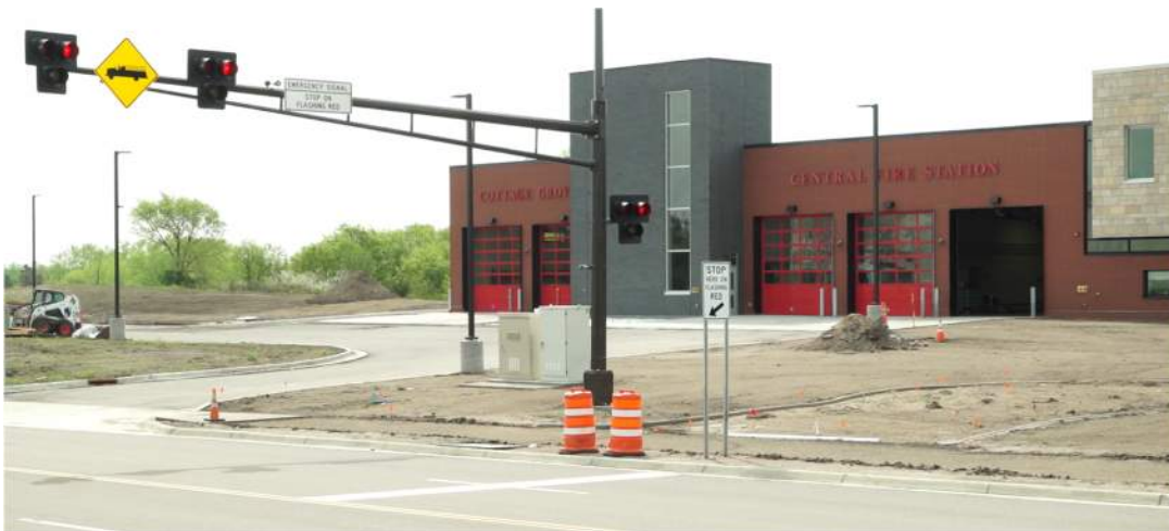
Figure 13: Emergency Vehicle Hybrid Beacon in Cottage Grove
