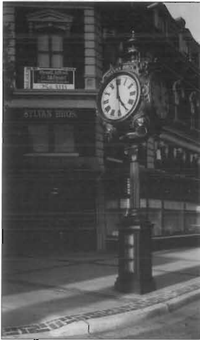
Photo: Jack E. Boucher, HABS.
