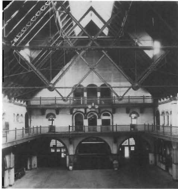
The exposed metal roof-truss system of this waiting room not only provides structural support, but is also important in defining the interior character of the train station.
