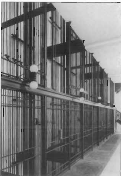
Both function and design elegance are evident in this row of cast iron elevator cages and light fixtures adorning an early-20th century commercial building.
