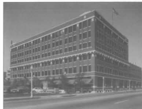
When the six-over-six windows were replaced with inappropriate single sheets of tinted glass, the historic industrial character of this building was lost.
