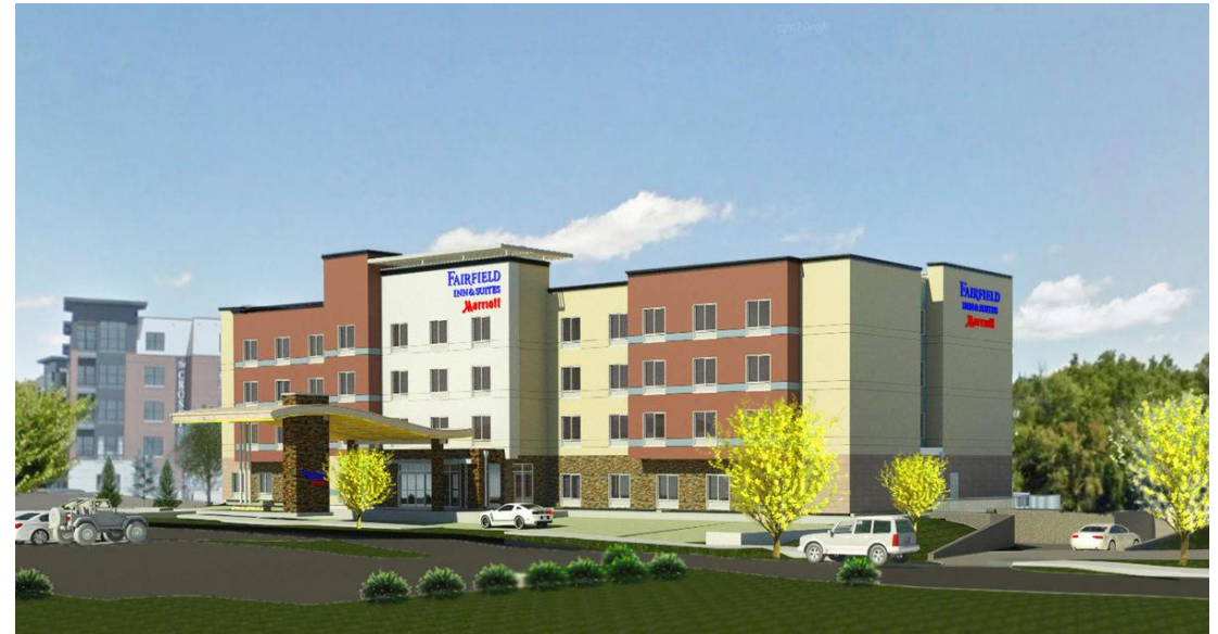
Fairfield Inn & Suites – Opened October 2018
