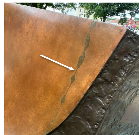
Figure 3. Visible, original weld on copper sheet
