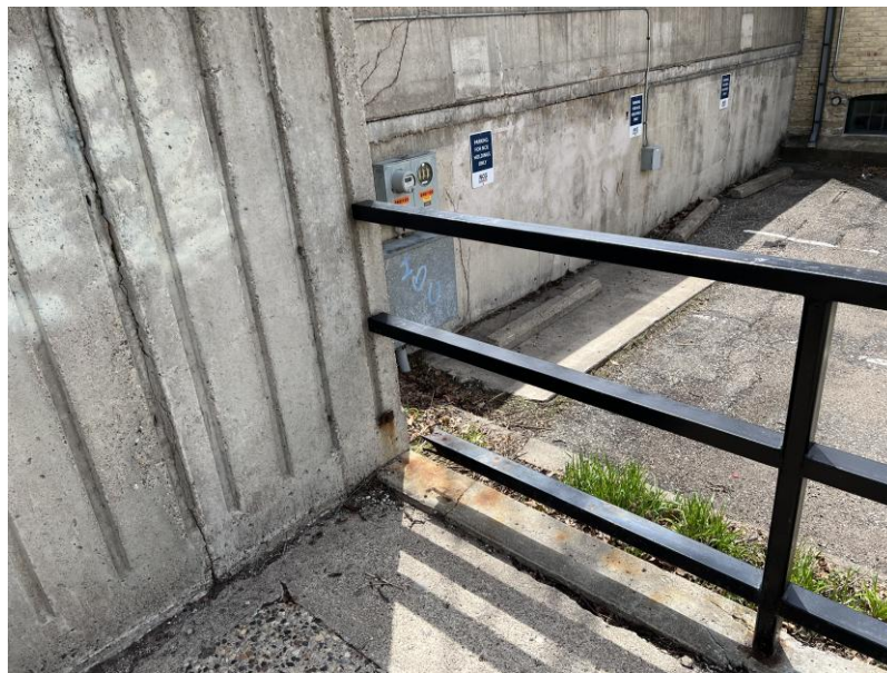
Broken railing
