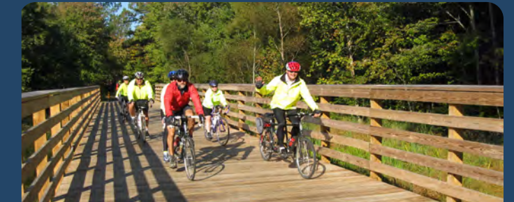
Where possible, use boardwalks and bridges to add interest and allow for intimate and unique river experiences.
