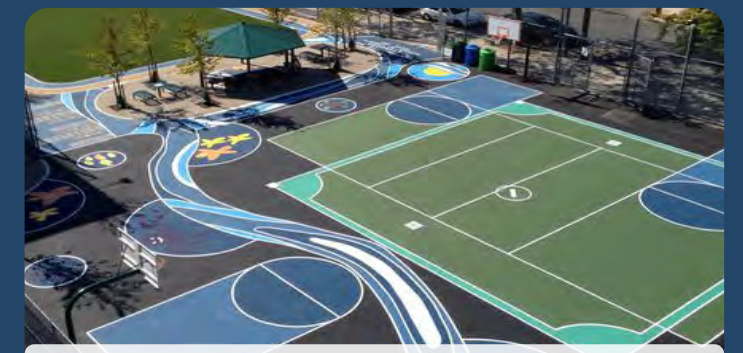
Construct state-of-the-art, multi-use game courts
