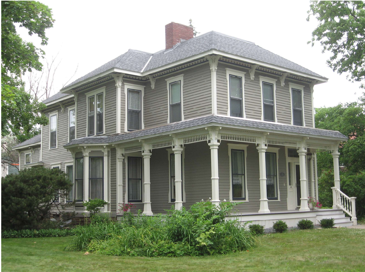
Current Photo (after 2007 removal of asbestos siding, reconstruction of porch, and painting). See photos of each side and close-up details on following pages.
