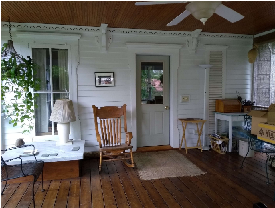
1998 screened in porch addition using existing doorway. Retained original cornice, corbels, moulded trim and wooden floor-to-ceiling slat vent (interior room was originally a fruit and vegetable bin).
