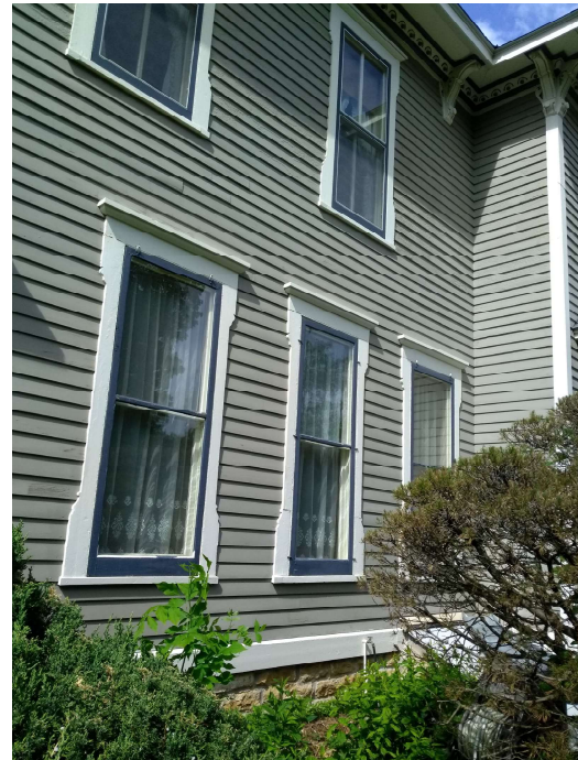
Early 1900s conversion of the doorway into a center window.
