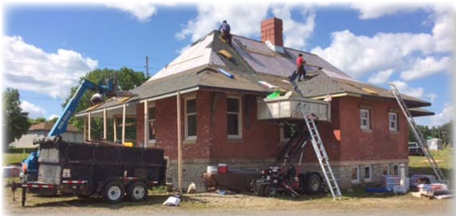
New Shingles: Spots on the roof were repaired before adding new shingles (donated by SageGlass/Saint-Gobain and their CertainTeed Roofing company). After shingling, interior work (e.g., insulation and drywall) could continue without threat of water damage.
