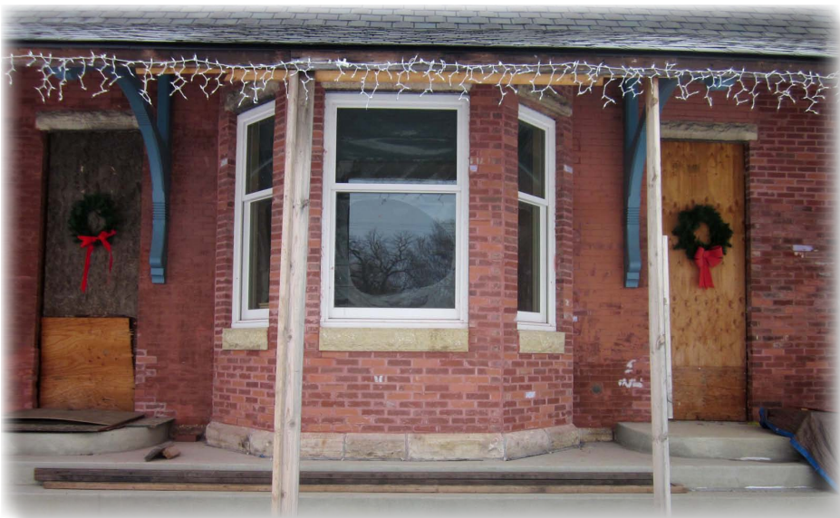
Station master's bay: A stone mason added reclaimed bricks, limestone water table and lintels to the station master bay constructed last year. Construction of the bay was funded with a donation by Norman and Lori Oberto and family.
