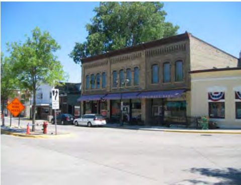
Existing view of historic building along Water Street
