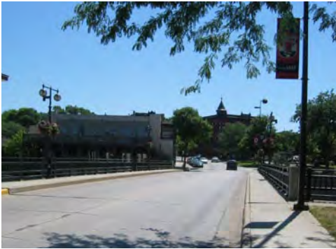
Existing view Water Street Bridge to Division Street
