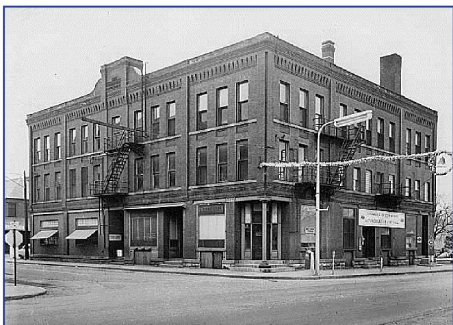
Lumbermen's Exchange, 101 S. Water Street (1890). MNHS
