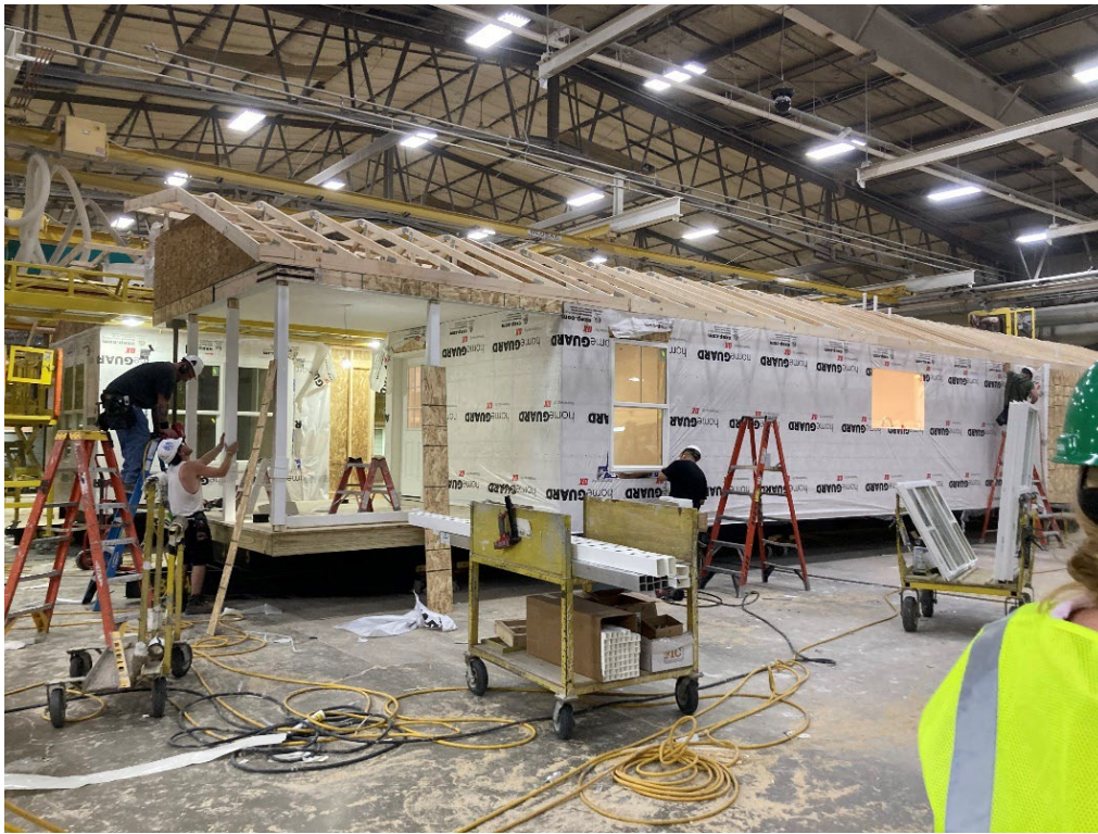
Schult manufactured home in the process of being built inside the factory
