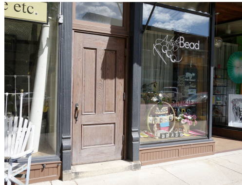
Central entry with cast-iron columns, 2016.
