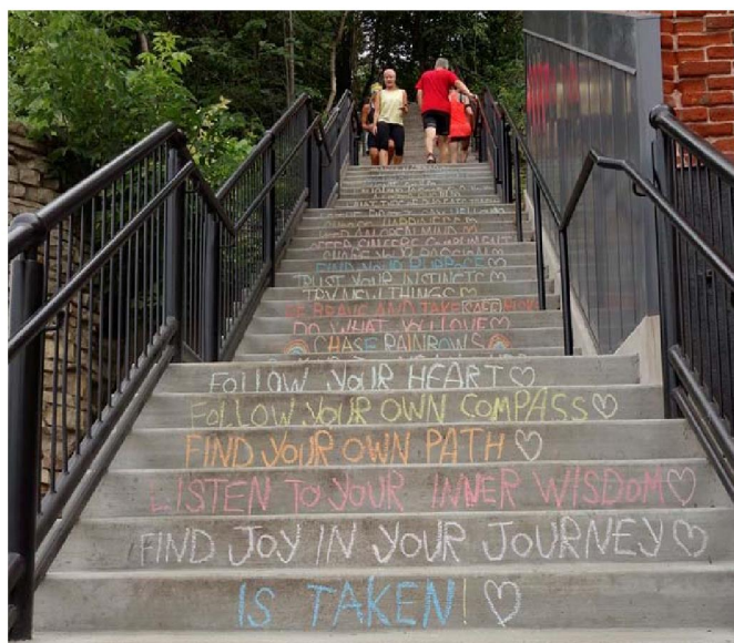
Public stairway reconstruction accompanied the adaptive reuse of the Joseph Wolf Brewery, 2018.
