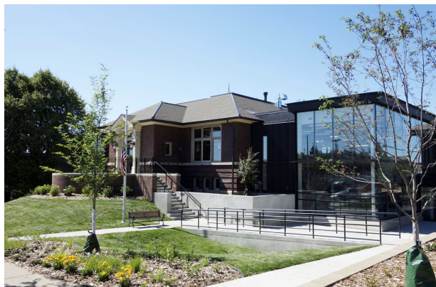
2016, looking northwest at new addition
