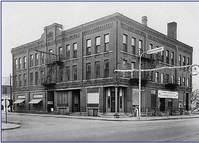
Lumbermen's Exchange, 101 S. Water Street (1890). MNHS
