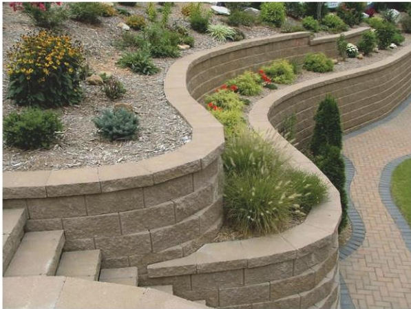
Figure 3-12: Retaining walls shall be benched, or terraced, so that no individual wall exceeds a height of six feet.
