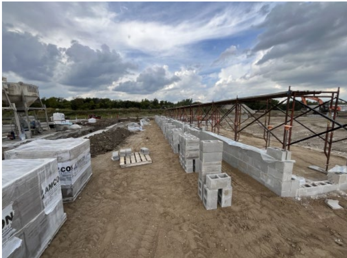
Stadia concrete blocks wall erection
