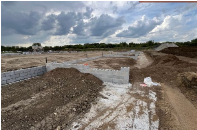
Stadia concrete blocks wall erection
