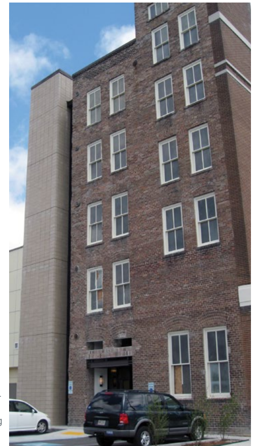
[62] The stair tower at the rear of this commercial building is a compatible new addition.
