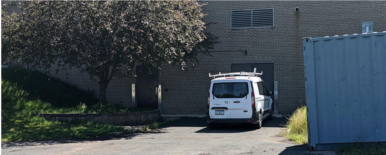
Figure 5-5 West Gym Doors
