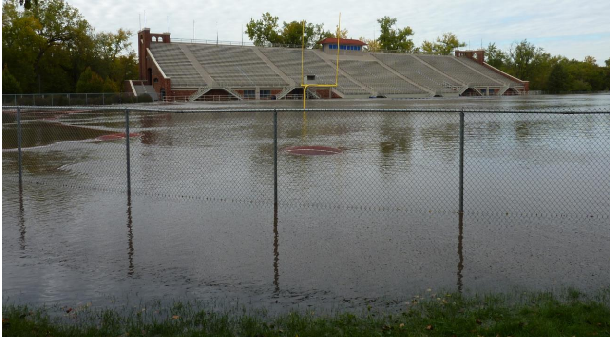
Figure 5-2 Stadium Flooding September 25, 2010
