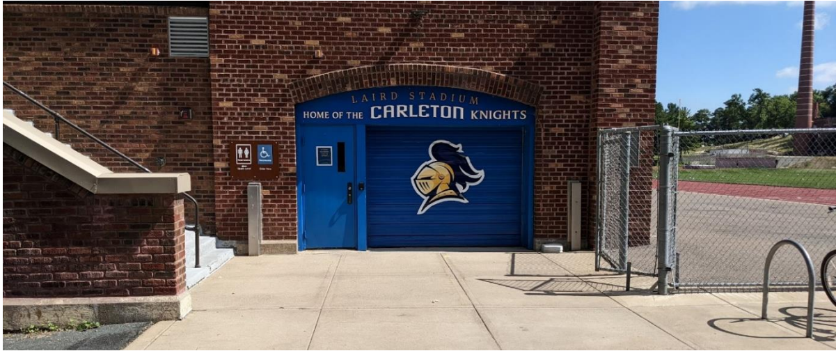
Figure 5-3 Stadium South Entrance with Posts for Stoplog Temporary Closure
