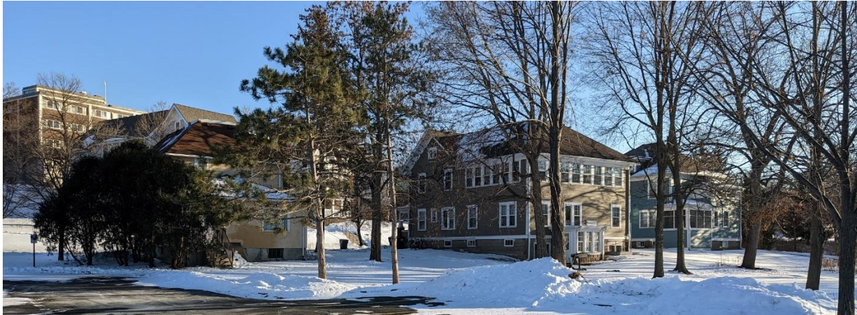
Figure 5-1 Student Houses (left to right: Wilson House, Allen House, Prentice House)
