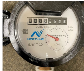
Water meter replacement
