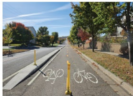
On-street cycle track along Maple St
