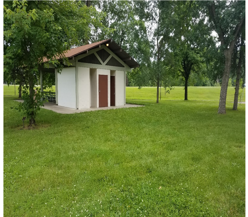
Install Sidewalk To Shelter
