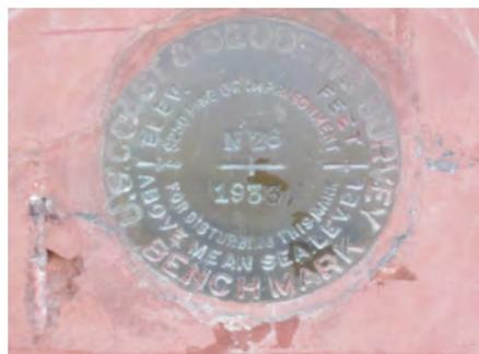
1933. Geodetic Elevation Disk installed in depot west wall, one of three in Northfield at the time to assist in planning developments. Decommissioned after depot move. National Geodetic Survey has requested to install a new, additional disk in current depot location.
