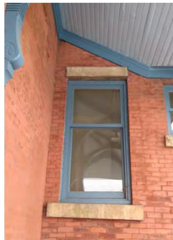
One of two 1910 windows with smooth concrete lintels and sills in the added restrooms in the former baggage room.
