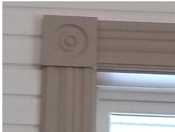
Above photos include original v-board, window and door casing, milled plinths and baseboard, and the newly crafted rosettes. Some of the elements were hand crafted because of the width needed for the casing. Fortunately, symmetrical casing of the width needed was available for purchase and being discontinued, and there was enough for the depot work. The width of all elements was consistent with the width of the shadows of the original.
