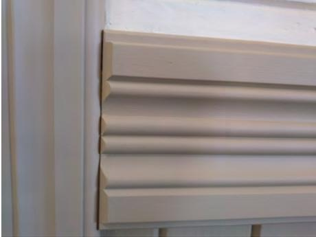
The wainscoting trim was milled to the width of the unpainted shadow found on the v-board wall. The profile used is very similar to that of the pieces of original casing found in the attic.
