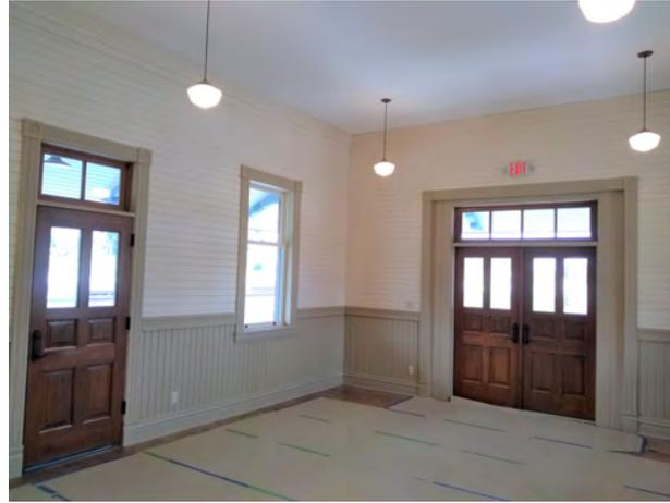
Evidence of the colors used in the interior were gathered from the original existing v-boards (chipped paint and nail holes from the plaster board) and pieces of the casing found in the attic.
