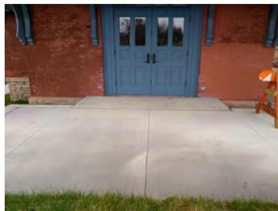
Connecting platform between depot double door and pavilion. Future ramp will be on the west edge of the pavilion (track side to the right). Top of water table visible in gap between platform and wall.
