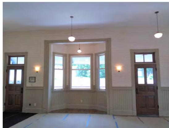
2019. Turned the two 1944 windows back into doors as in 1888; restored the 1888 station master bay and installed cottage windows.
