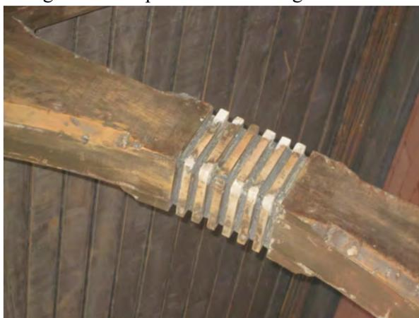
Repair: Some corners of bracket slots were missing, but repaired. Nail holes were filled. Wood in excellent condition.
