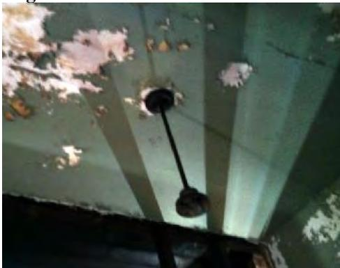
One pendant light fixture was found in the original ceiling of the baggage room area. The ceiling had never been removed and lowered, in contrast to the main room.
