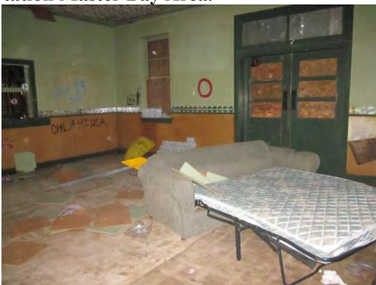
2016. 1944 remodeling converted a door into the window (left); removed the station master bay and replaced with a double door.
