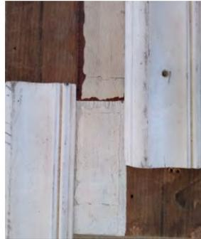
Mock up of crown moulding placing two pieces of moulding on each side of the 7” board.
