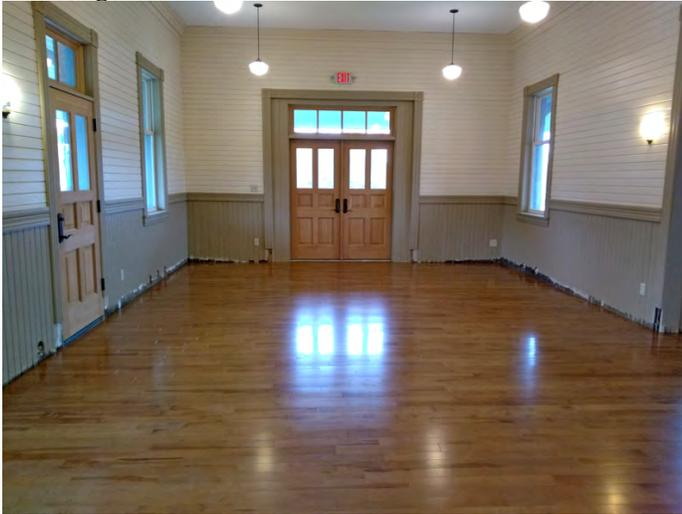
The 1888 maple flooring was covered with concrete and rubber tile in the 1944 remodeling. That work included the removal of the dividing walls around which the original flooring had likely been laid.
