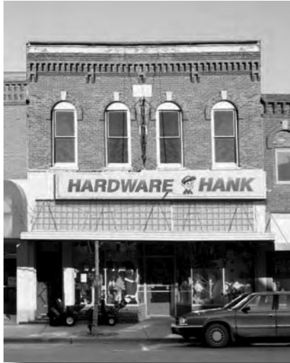
Backlit plastic signs and underlit awnings with lettering are inappropriate for historic buildings.
