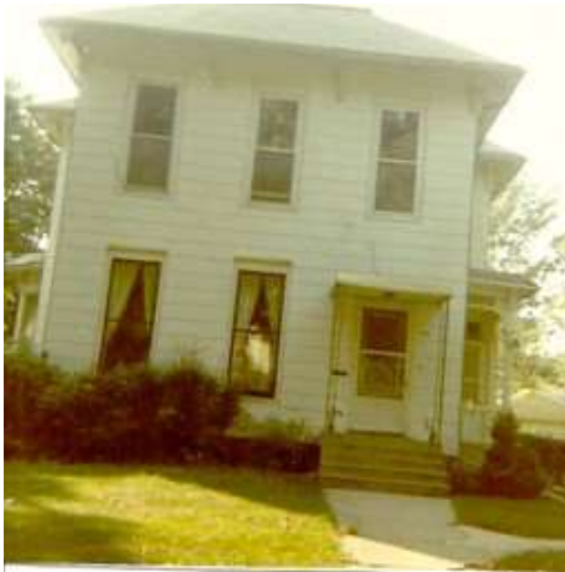
Before restoration: Original porch removed in the 1950s and replaced with concrete slab steps; variegated metal roof and wrought iron posts; exposed electrical wire for porch light.
