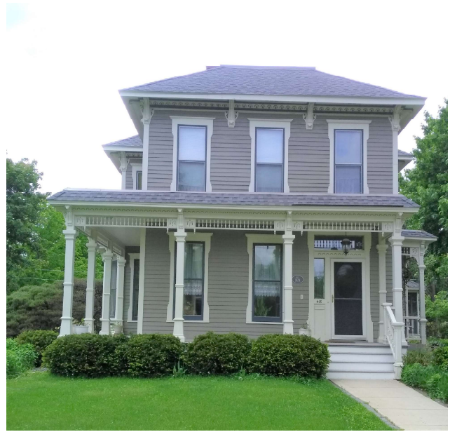
After restoration: Porch restored with original height, size and style of pillars, size and style of doorway, decorative spanner and corbels to match those on the original side porch on right.
