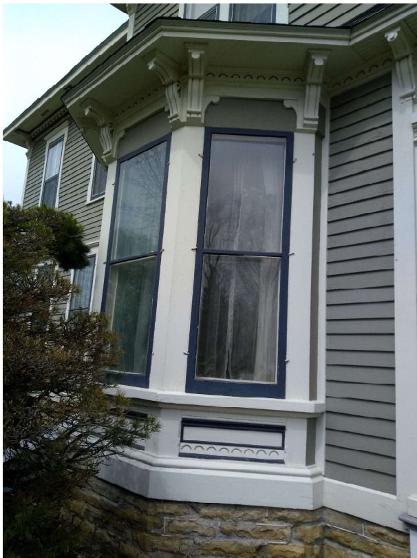
Side bay windows; insert wooden panels in bay. All original wood including storm windows with old glass. The original brackets on this bay were used to replicate the brackets on the reconstructed porch in photos above.
