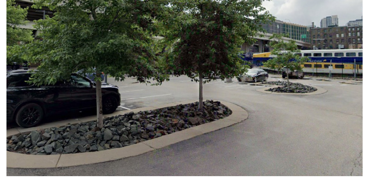
stormwater trench
