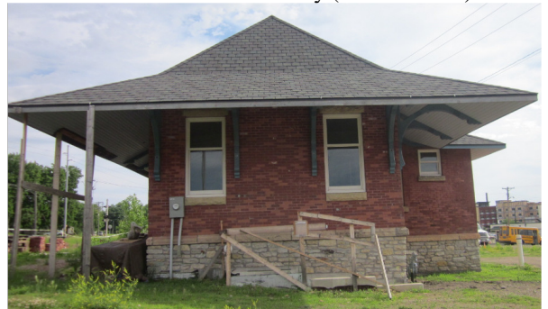
West side (track side): red arrows = 1944 windows added in 1888 door openings (now restored); yellow arrow = 1944 addition of doors after removal of 1888 station master bay (now restored).
