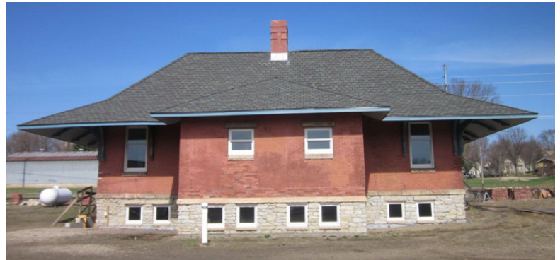
East side (Hwy. #3): Reflects 1911 bump-out modification of baggage room into bathrooms and boiler room.
