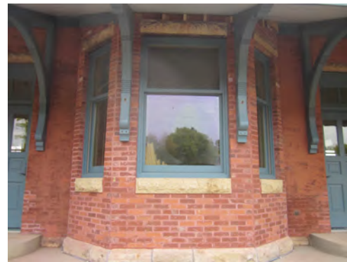
2019 Reconstructed station master bay
