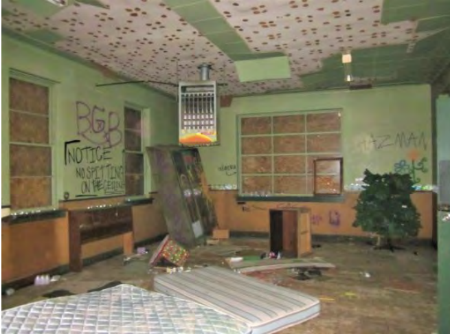
2016: Reflects 1944 changes: Ceiling lowered 2 ft.; acoustical tile used. Note also, all woodwork removed; 1” of plaster added over wood walls; windows replaced; concrete & tile added on top of wood floor.
