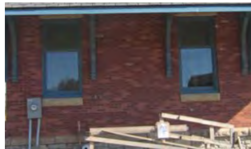
2019 South wall with added recycled brick
