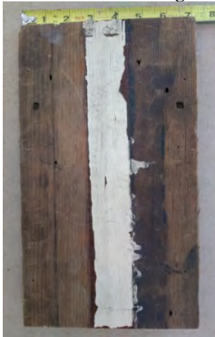
2016: Crown moulding component found in attic
