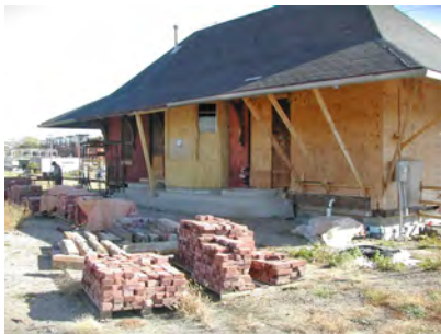
2017 New walls needing brick
