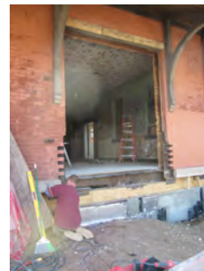
2019 Retained location of 1944 opening, lintel and brackets.
