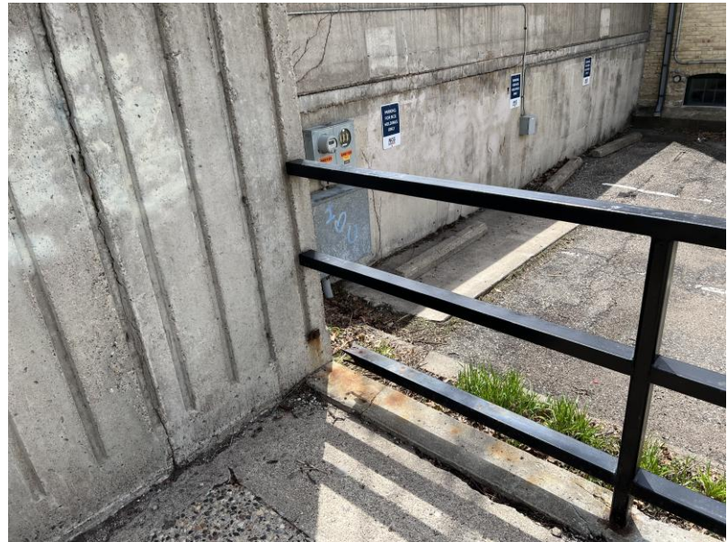
Broken railing
