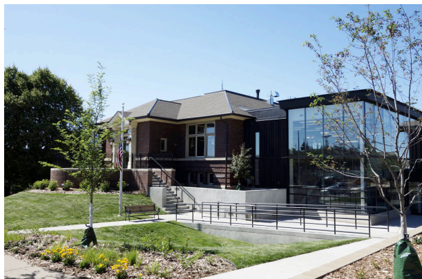
2016, looking northwest at new addition
