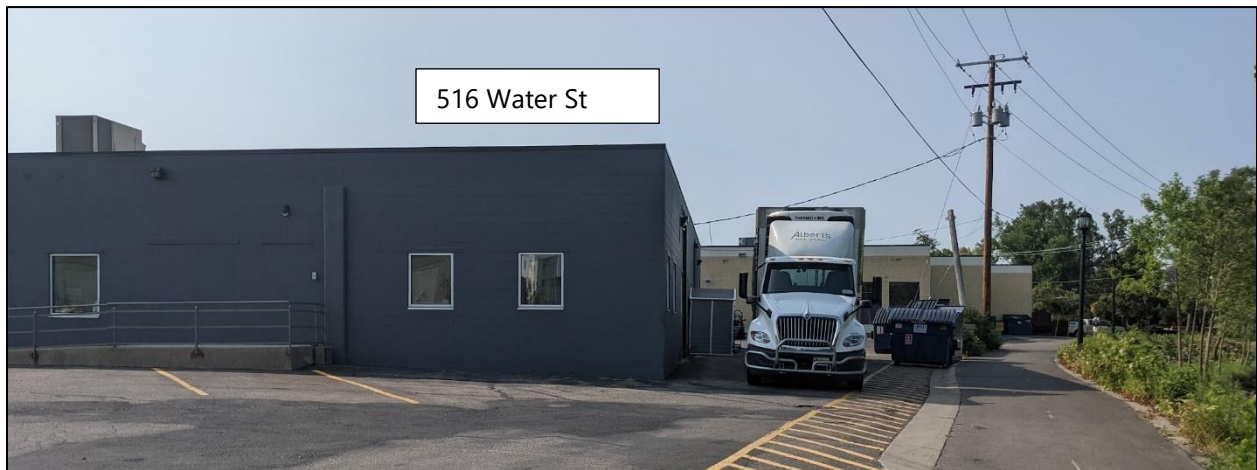
Figure 4-7 Just Food Co-Op Building Looking South
