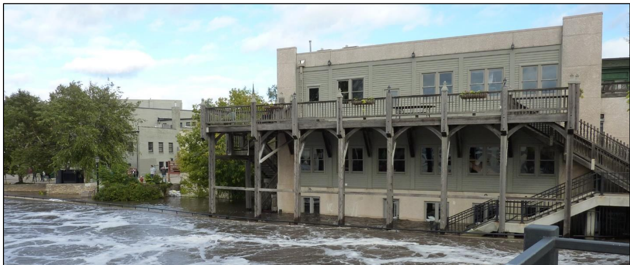
Figure 4-5 Cannon River Overflowing Channel Wall at 11 Bridge Square September 24, 2010
