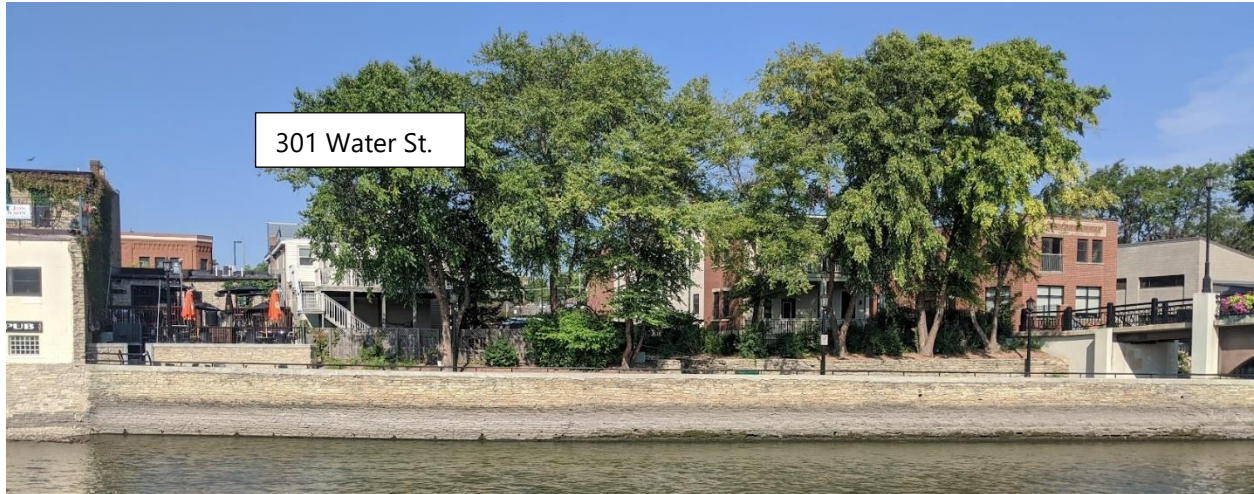
Figure 4-1 West Bank Riverwalk Properties Upstream of Pedestrian Bridge
