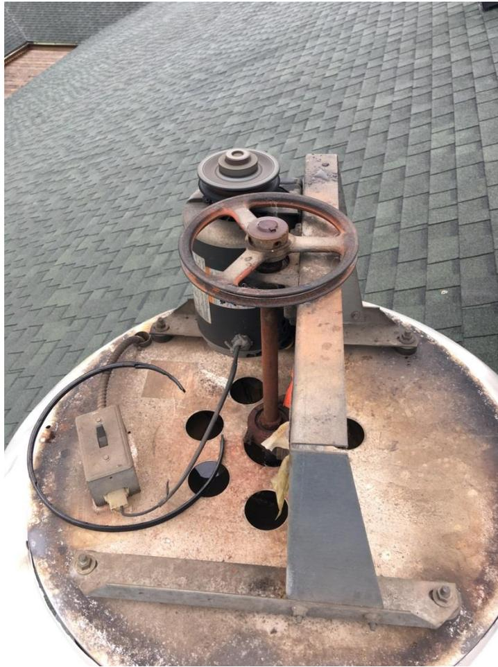
PICTURE OF LOCKER ROOM EXHAUST FAN; Motor is spinning, fan does not move well as bearings appeared to be in poor condition, belt was worn and broken.
