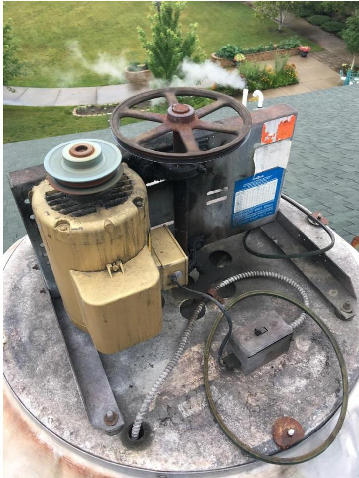
PICTURE OF POOL EXHAUST FAN UNIT; Belt is off, but motor is spinning.
