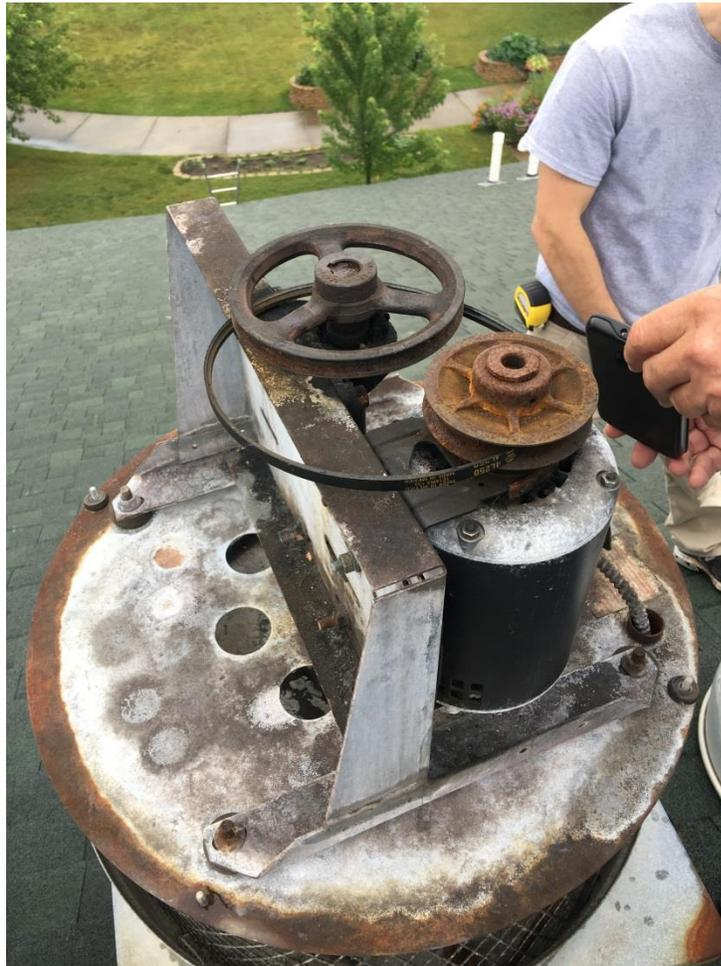
PICTURE OF JACUZZI EXHAUST FAN; Both the fan and the motor are seized.
