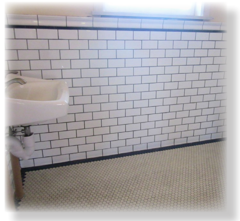
The accessible restroom was tiled, and fixtures were installed this year.
