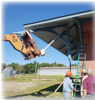
The two new corner brackets crafted this year were so large and heavy that a forklift was required for installation.
