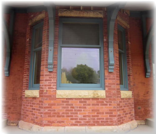
The last two new brackets to be crafted and installed were the small brackets on the reconstructed station master bay; the original bay was removed in the 1944 remodeling.
