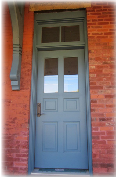
The doors and transoms were custom ordered using the original 1888 blueprint design; the double doors will open onto the floor of the pavilion.
