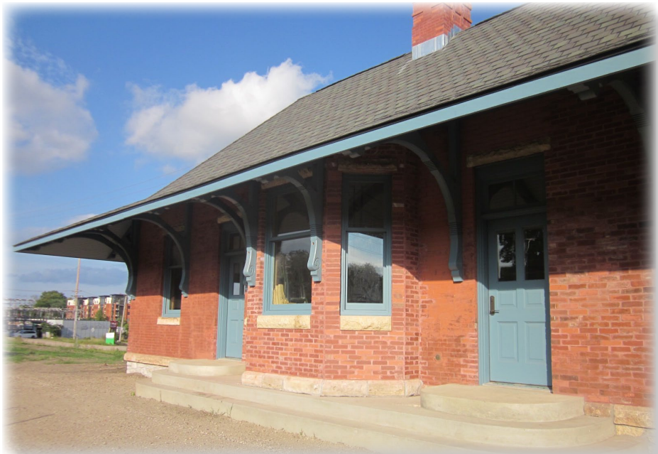
The depot's restored exterior
