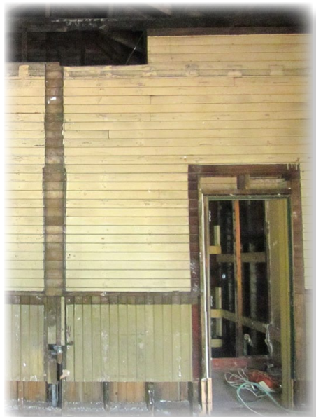
Volunteers removing one inch of plaster to reveal V-groove board on original wall and wainscoting
