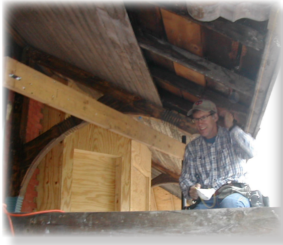
Volunteer carpenter repairing a soffit
