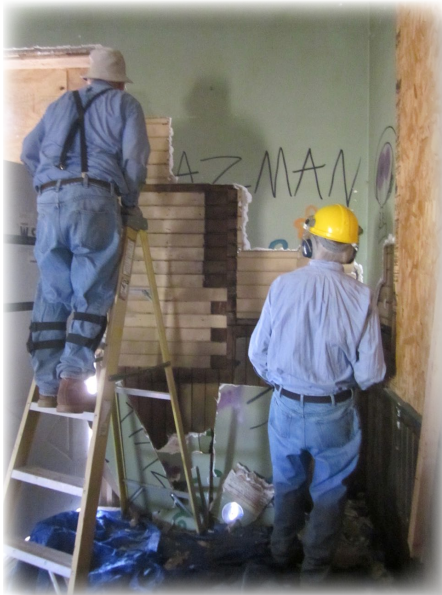
Volunteers removing one inch of plaster to reveal V-groove board on original wall and wainscoting
